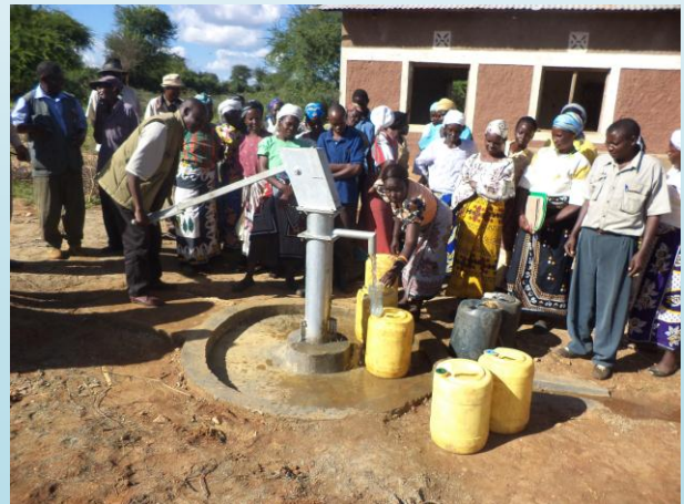
Completed Borehole at Nguni
