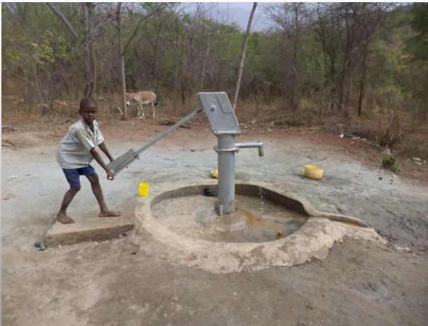
Completed Borehole at Ikongo
