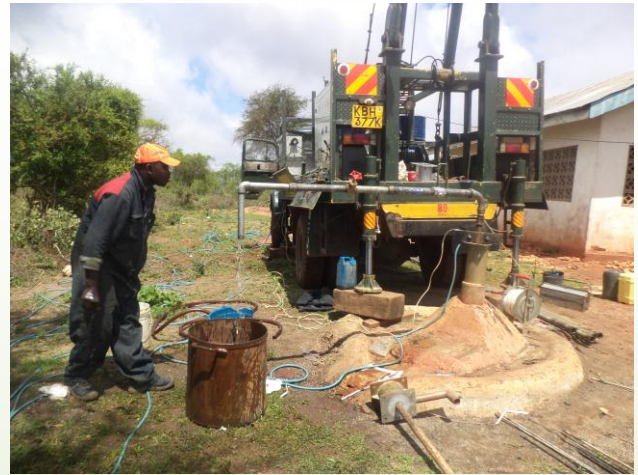
Removal of Broken Pipes & Recharge Testing by Kisima Drilling E.A
