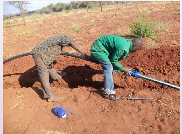
Laying of 2" PVC Pipes
