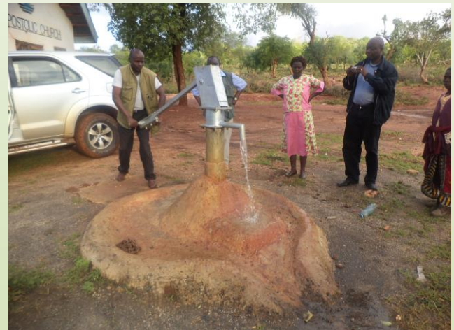
New Hand Pump Was Installed
