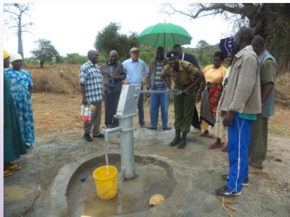
Completed Borehole at Katse
