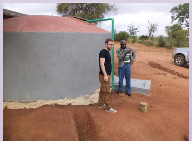
This Tank Was also Rehabilitated
