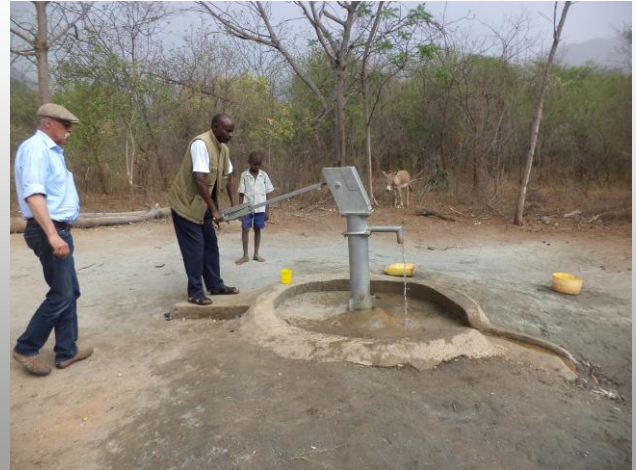
Completed Borehole at Ikongo
