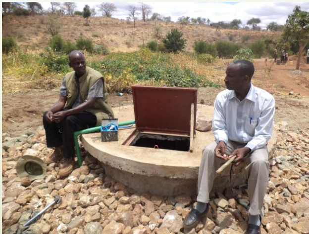
The well is sealed & Installed with a Submersible Pump
