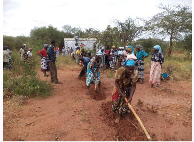
The Community Dug the Trenches
