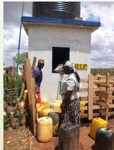
Water Kiosk Completed
