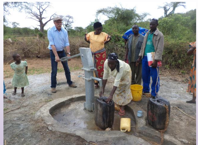
Completed Borehole at Katse
