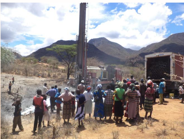
Drilling Started by Kisima Drilling EA Ltd
