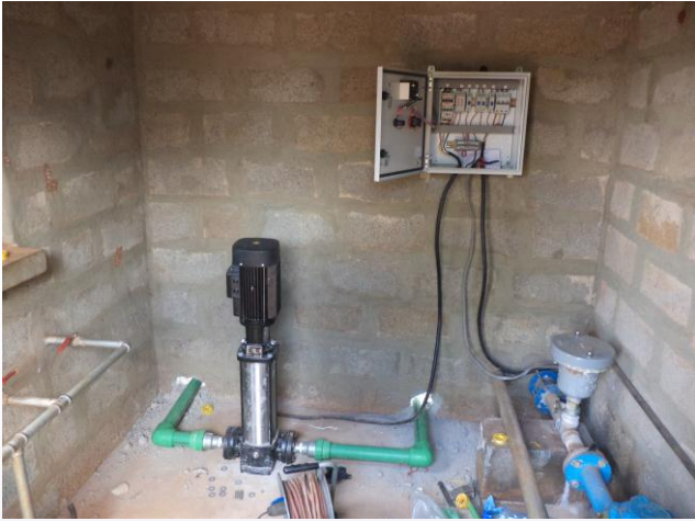
Installation of Grundfos CR 5-16 Pump
