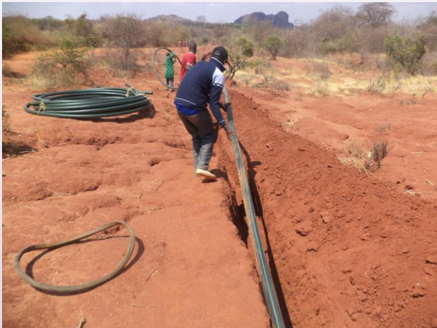
Laying of 2" PVC Pipes
