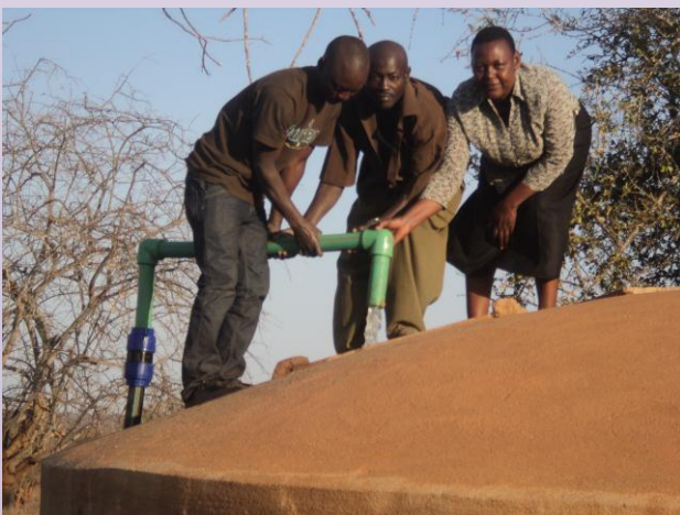
Pump Testing at Ndathani School
