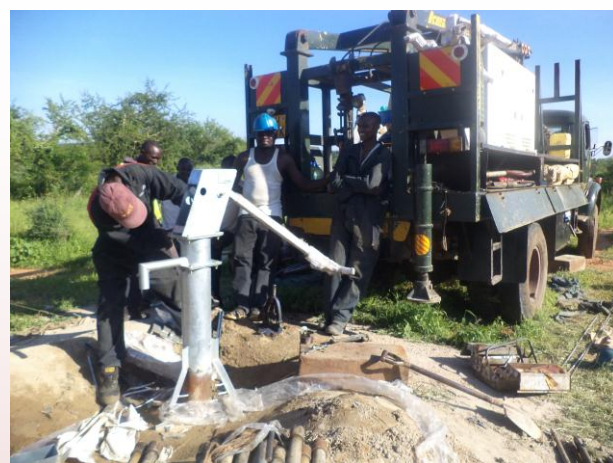
Pump Installation & Recharge Testing
