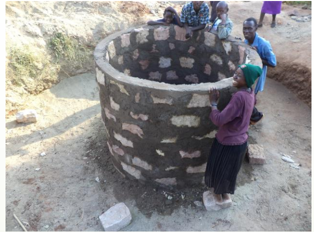
The Well is completed
