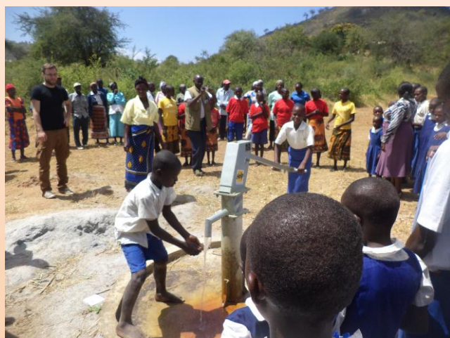
Completed Borehole at Thua
