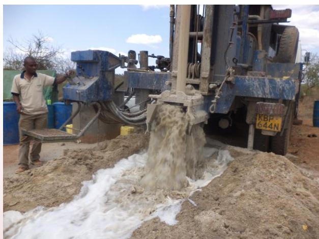
Drilling by Testek Water Services
