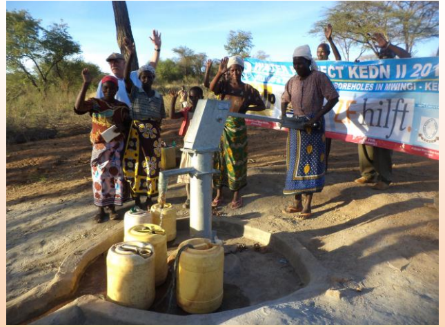
Completed Borehole at Waita
