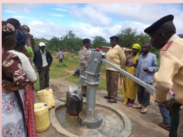
Completed Borehole at Ndiuni
