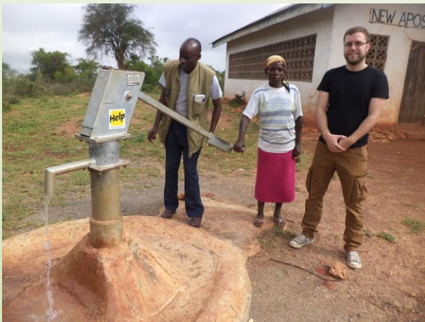
New Hand Pump Was Installed
