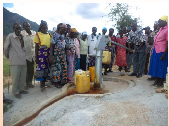
Completed Borehole at Mukonga
