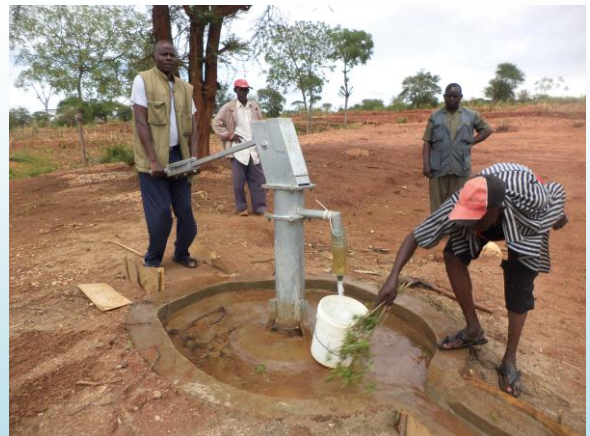
Completed borehole at Mutanda
