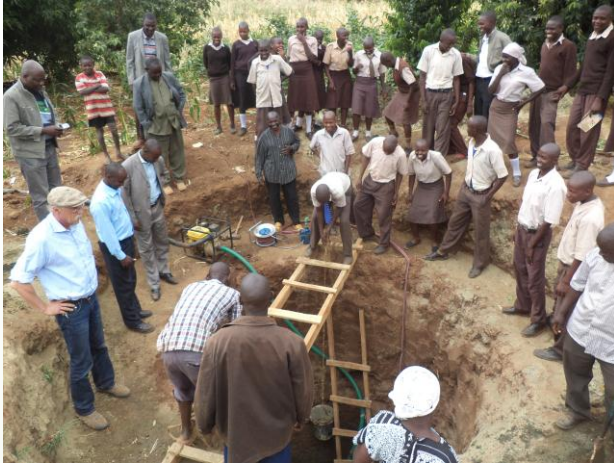
Community Started by Digging the Well
