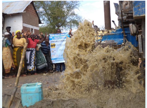
Borehole Undergoing Development
