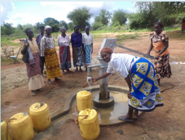
Completed Borehole at Nguni
