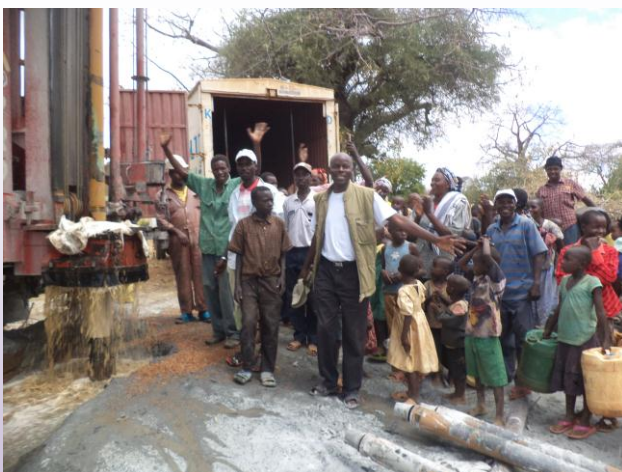
Kisima Drilling Strikes Water at Katse
