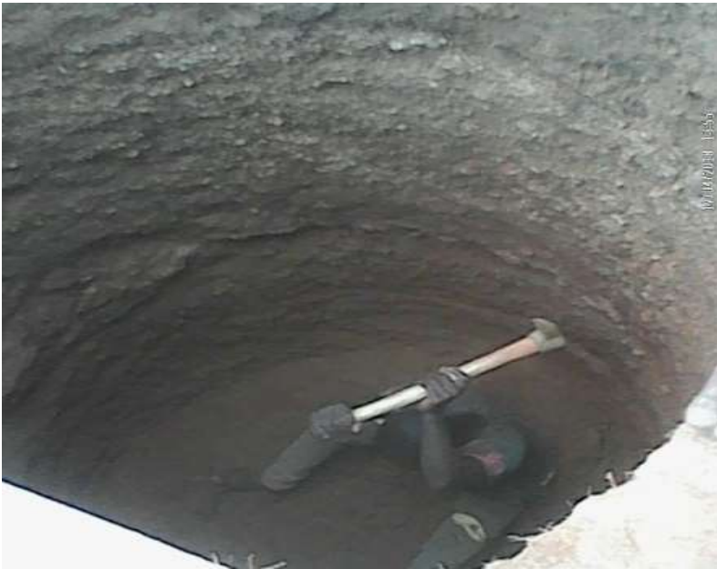
FIGURE 4: DIGGING OF THE BORE HOLE STARTS
