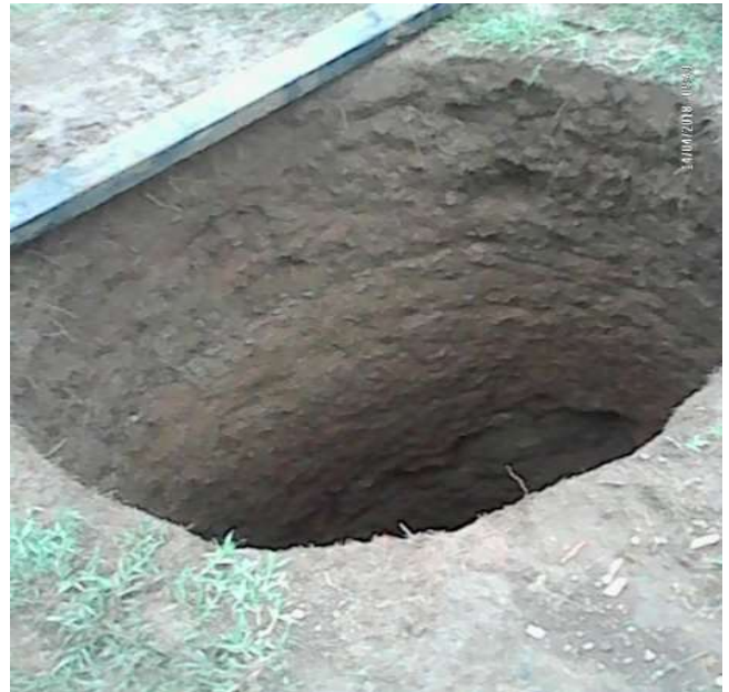
FIGURE 5: THE ROCK WAS FOUND JUST AFTER 5 FEET OF DIGGING
