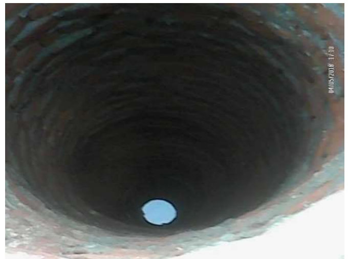
FIGURE 7: THE WATER HAS FINALLY BEEN REACHED AFTER SEVERAL ATTEMPTS
