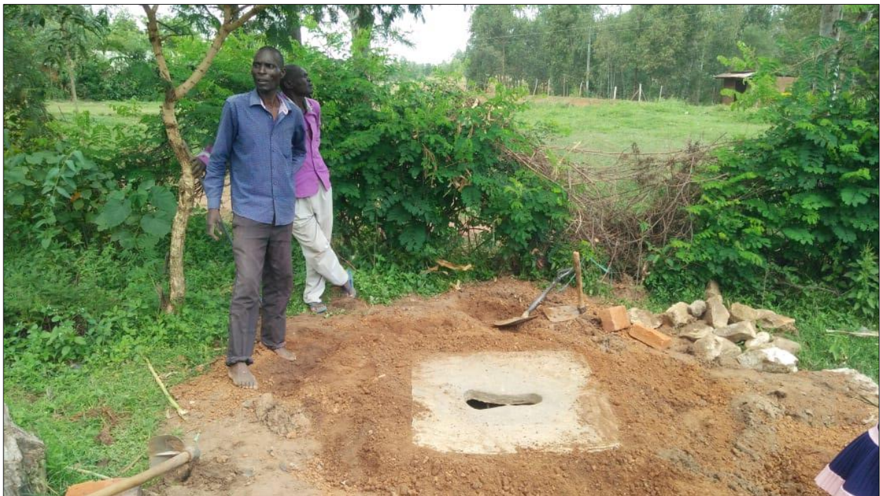
Arboloo/SANPLAT latrine under Construction-Slab Mounted on the pit latrine
