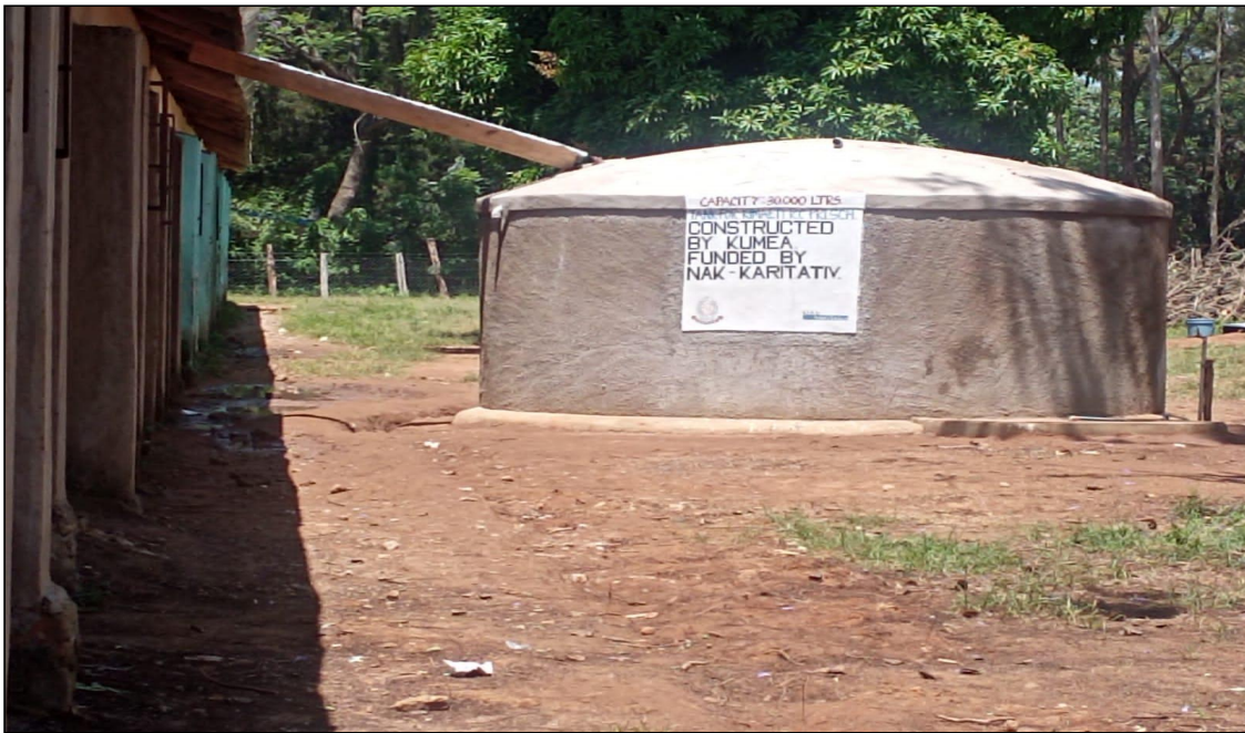
7.0 Completed 30,000litres Ferro-cement Water Tank for Kimaeti Primary Boarding &Day school
