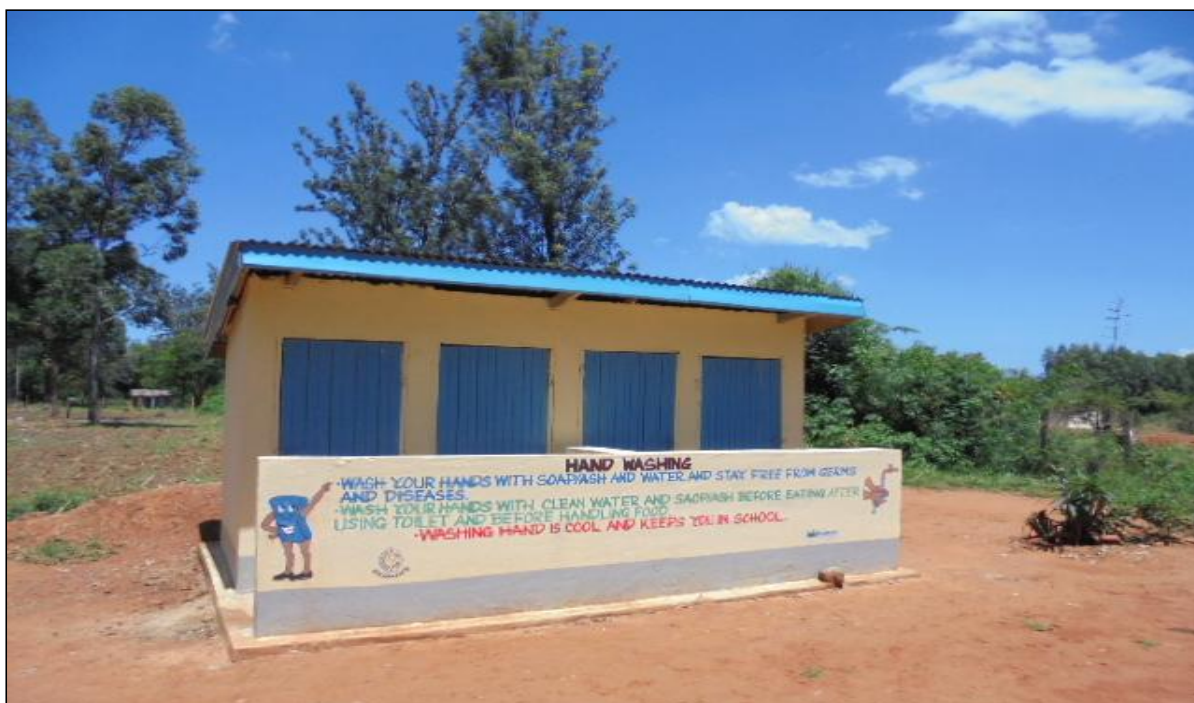
2.0 Completed 1no. 4door Ventilated Improved Pit latrines for Kimaeti Primary Boarding & day school
