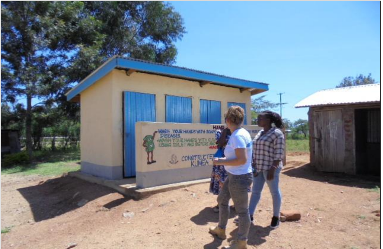
3.0 Completed 1no.4door Ventilated Improved Pit latrines for Shilila Primary School
