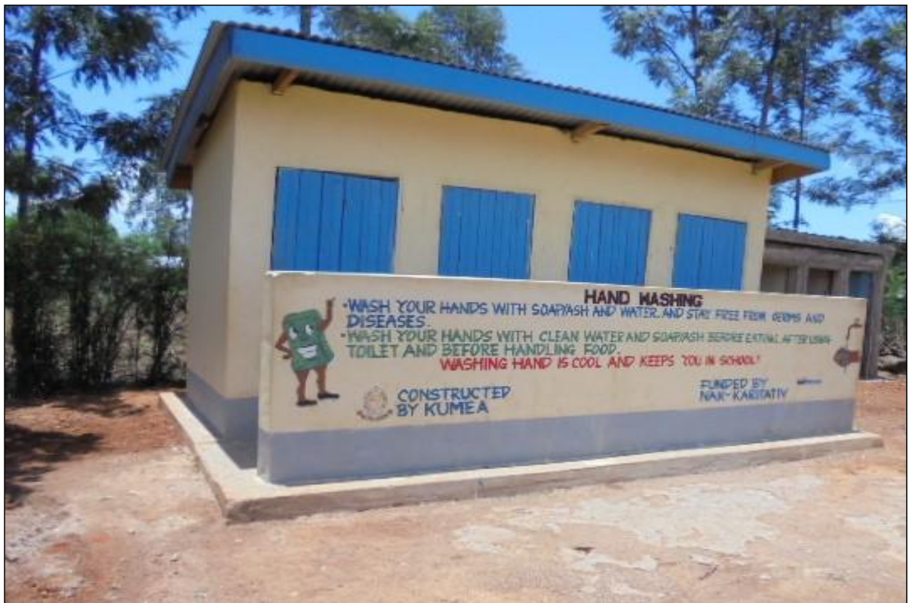
4.0 Completed 1no.4door Ventilated Improved Pit latrines for Nakalila Primary School
