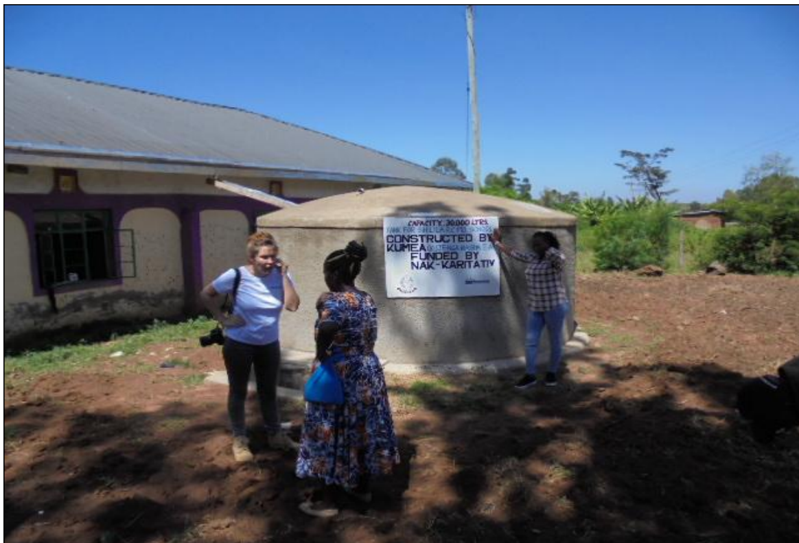
1.0 Completed 30,000litres Ferro-cement Water tank at Shilila Primary School
