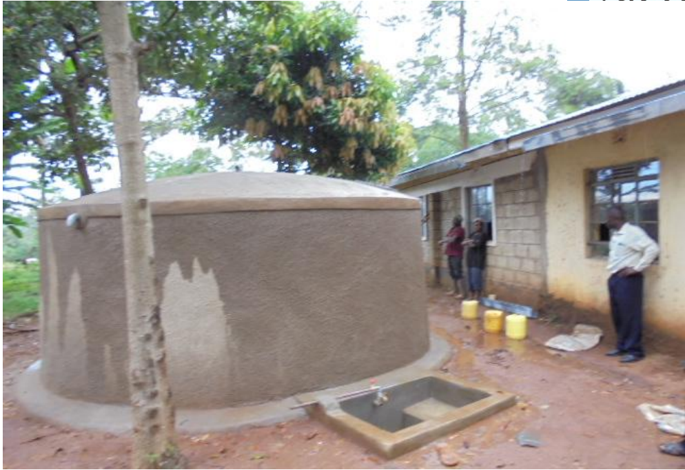
3.0 Completed 30,000 Ferro-cement water tank for Chandugunyi Primary School in South Maragoli location ,Vihiga Sub-county
