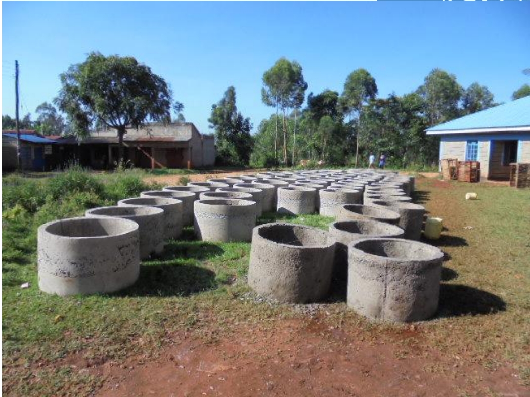
1.0 Culverts production for hand dug well construction at Ebukolo chief Office,Emuhaya sub-county
