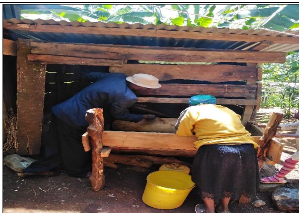
3. Inspection of the completed animal stable/pen for Kamanu Women group member
