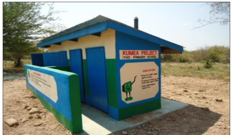
23. New VIP Latrines completed for Itiko Primary school in Kituyi County
