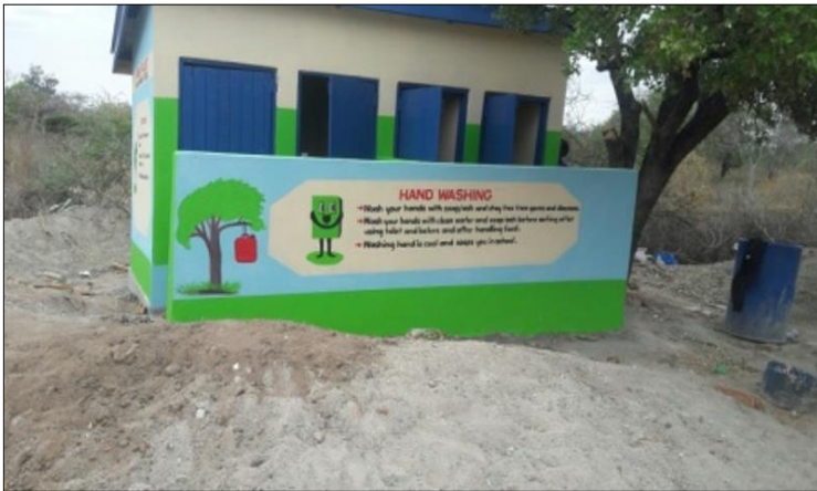
9. Completed VIP Latrines for Malatani Pri. School
