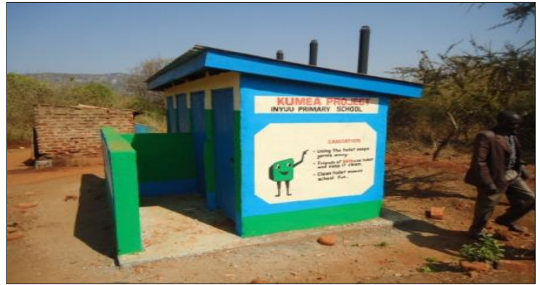
19. New VIP Latrines completed for Inyuu primary school in Kituyi County
