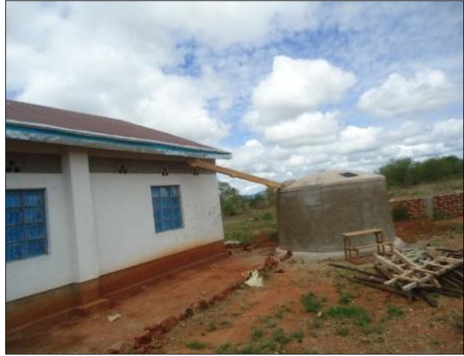
2. Matulani Sec. school Ferro-cement Water Tank
