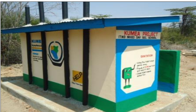
22. New VIP Latrines completed for Itiko mixed secondary school in Kituyi County
