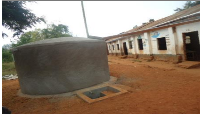
4. Completed 3 rd Ferro-cement tank for Kambu primary school.
