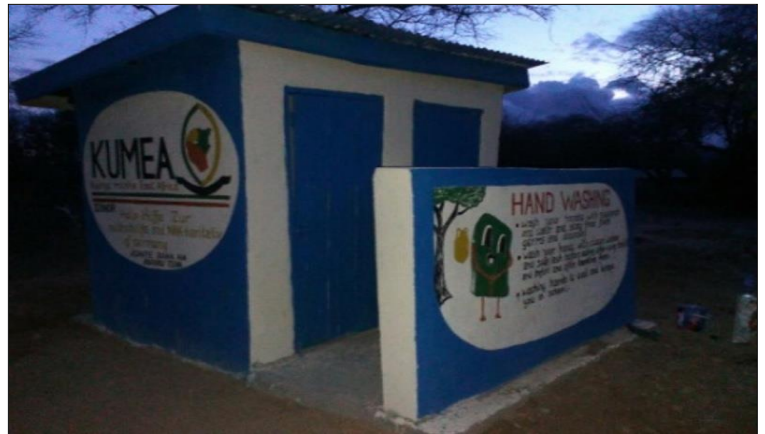
8. Completed VIP Latrine for Mangola Pri. School
