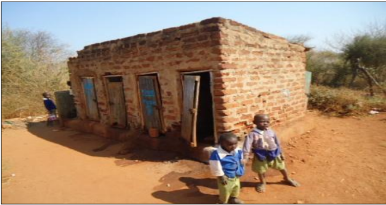
18. Old latrines for Inyuu primary school in Kituyi County
