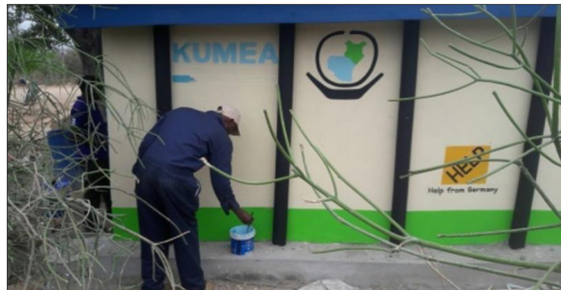
12. Completed VIP Latrines for Kavaani Pri. School
