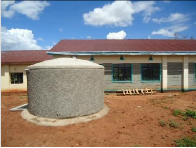
1. Nthongoni Sec. School Ferro-cement Water Tank
