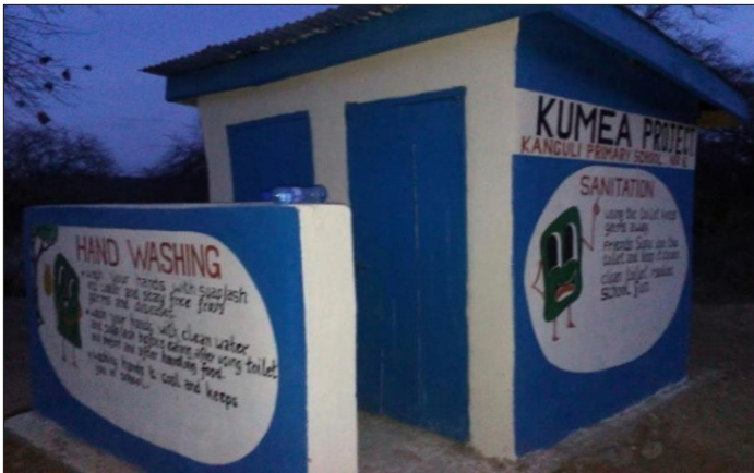
7. Completed VIP Latrine for Kanguli pri. School
