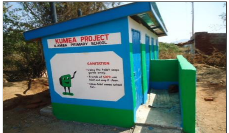
27. New VIP Latrines Completed for Ilamba primary school in Kituyi County
