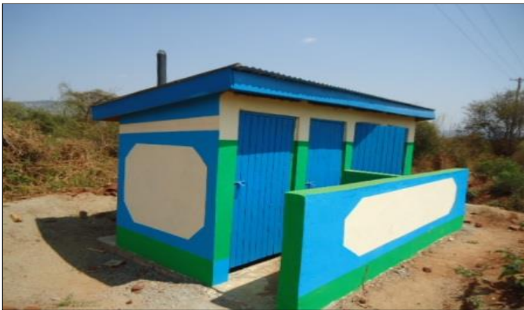
26. New VIP Latrines Completed for Kwa-ombe primary school
