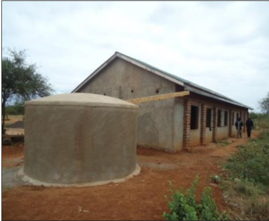
7. Completed ferro-cement tank at Kyaani P.School.
