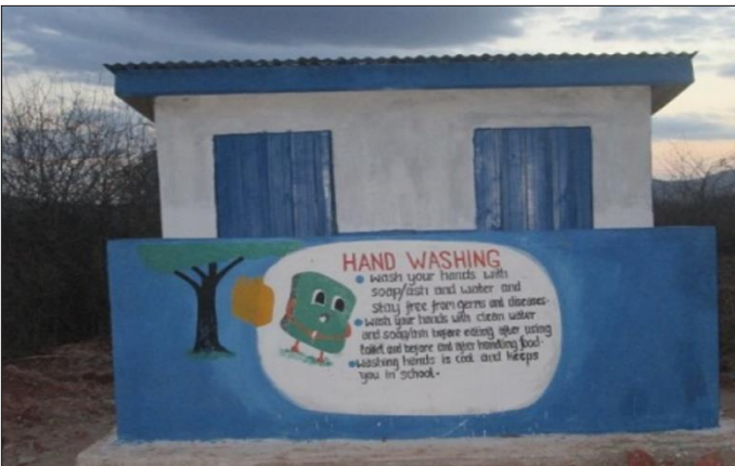
Photos 5-6: Completed and in use 1No. 2door VIP –Ventilated Improved Pit latrines for Hon Kiema Pri. School
