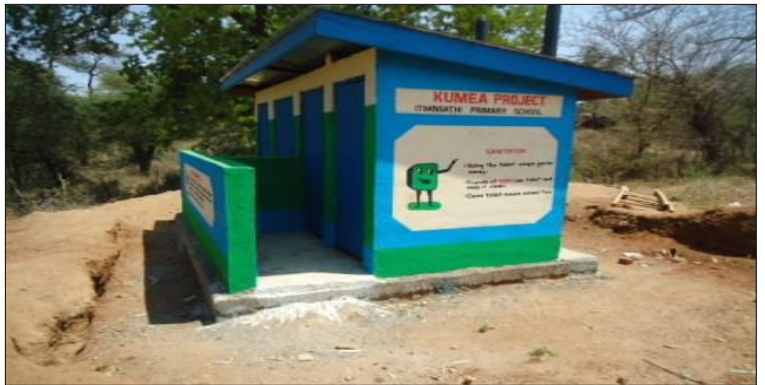
21. New VIP Latrines completed for Ithangati primary school in Kituyi County
