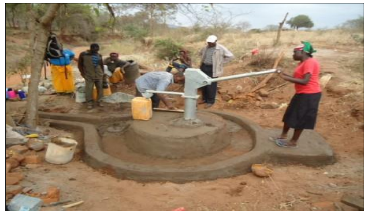
11. Completed Ferro-cement tank at Nzoila Sec. School
