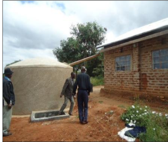
7. Completed ferro-cement tank at Kyaani P.School.
