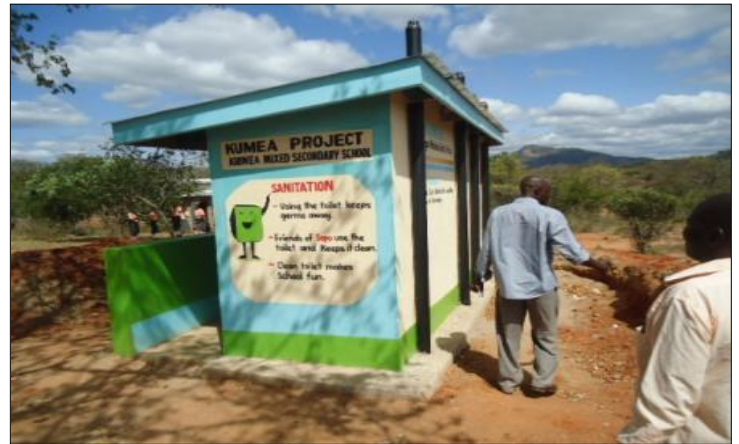
10. Completed VIP Latrines for Kibwea sec. school
