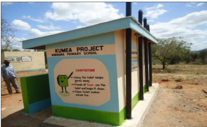
11. Completed VIP Latrines for Winduma Pri. School
