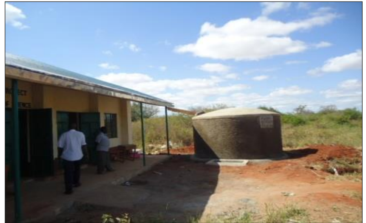
11. Completed Ferro-cement tank at Nzoila Sec. School
