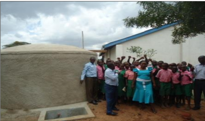
5. Thamba-Aume Pri.School Ferro-cement tank school
