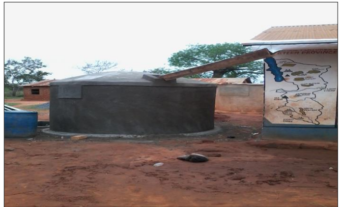
6. Completed 1 st Ferro-cement Tank for Kambu Pri.
