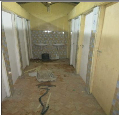
7. Works being completed from inside latrines
