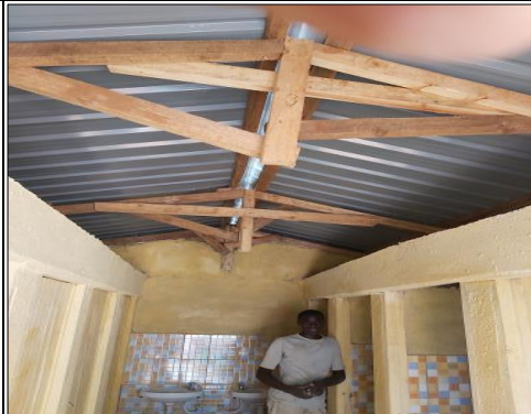
5. Inside the completed latrines
