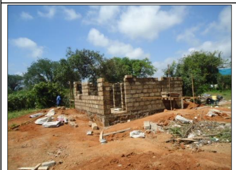
7. Latrine Construction works in progress at Kalulini High school
