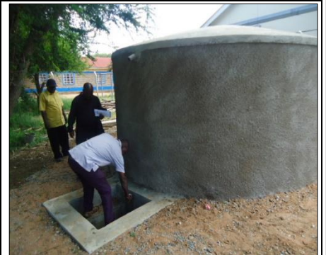
3. 1 st Completed Ferro-cement water tank of 30,000litres at Kalulini High school
