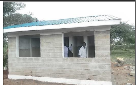
9. Inspection of Latrines construction works at Kalulini high school
