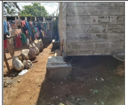
3. Latrines connected to chambers
