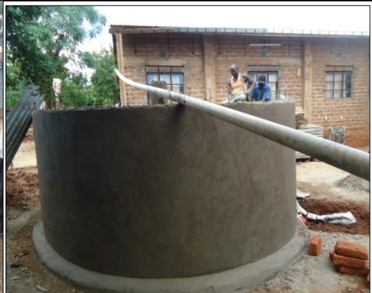
6. Ferro-cement water Tank construction works in progress at Kaundu secondary school
