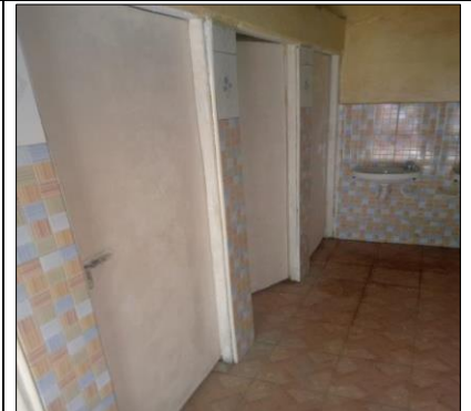
6. Inside view of the latrines
