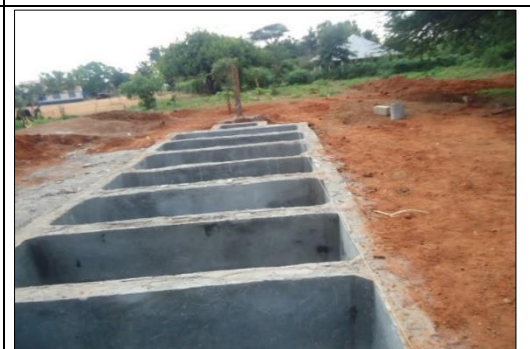
9. Construction works of the sludge chambers at Kalulini high school
