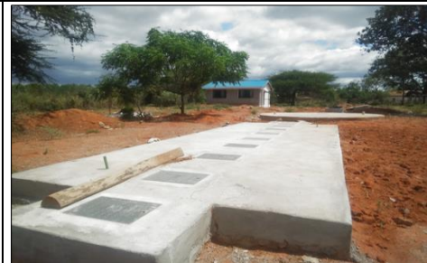
8. Sludge chamber for Biogas production completed at Kalulini High school
