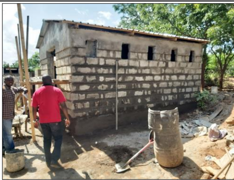
2.Rear view of the latrine's construction
