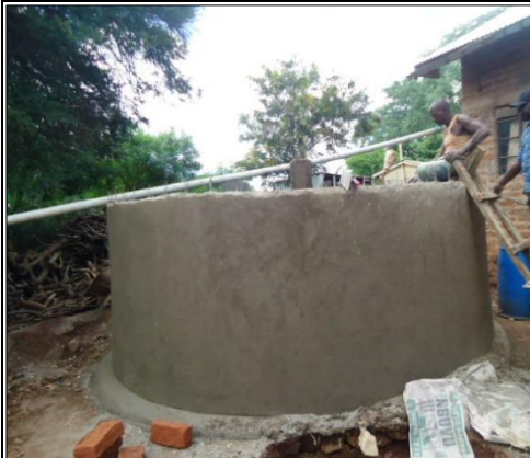
4. Ferro-cement tank construction works process at Kaundu secondary school
