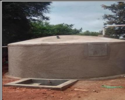
5. 1 st Completed Ferro-cement water tank of 30,000litres at Kaundu Secondary school
