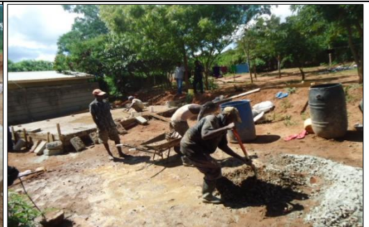
3. Commencement of latrine construction works at Kaundu secondary school
