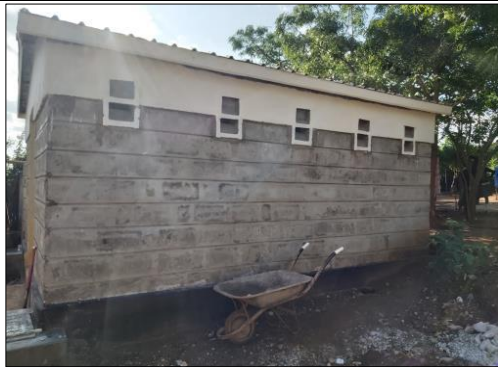
4. Completed rear view of the latrines
