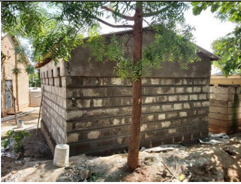
1.Side view of the latrine construction
