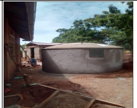
6. 2 nd Completed Ferro-cement water tank of 30,000litres at Kaundu secondary school
