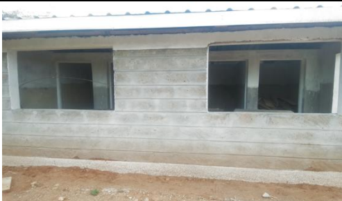
7. School latrines construction works on-going at Kalulini high school
