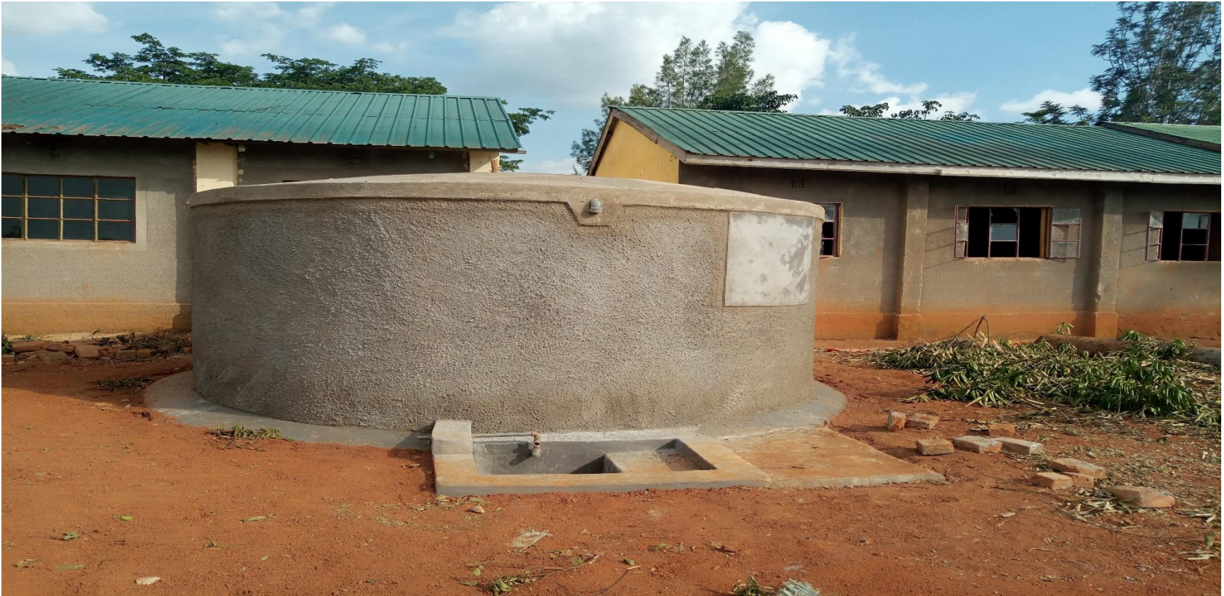
Complete ferro – tank at St. Moses Sigwata Primary School
