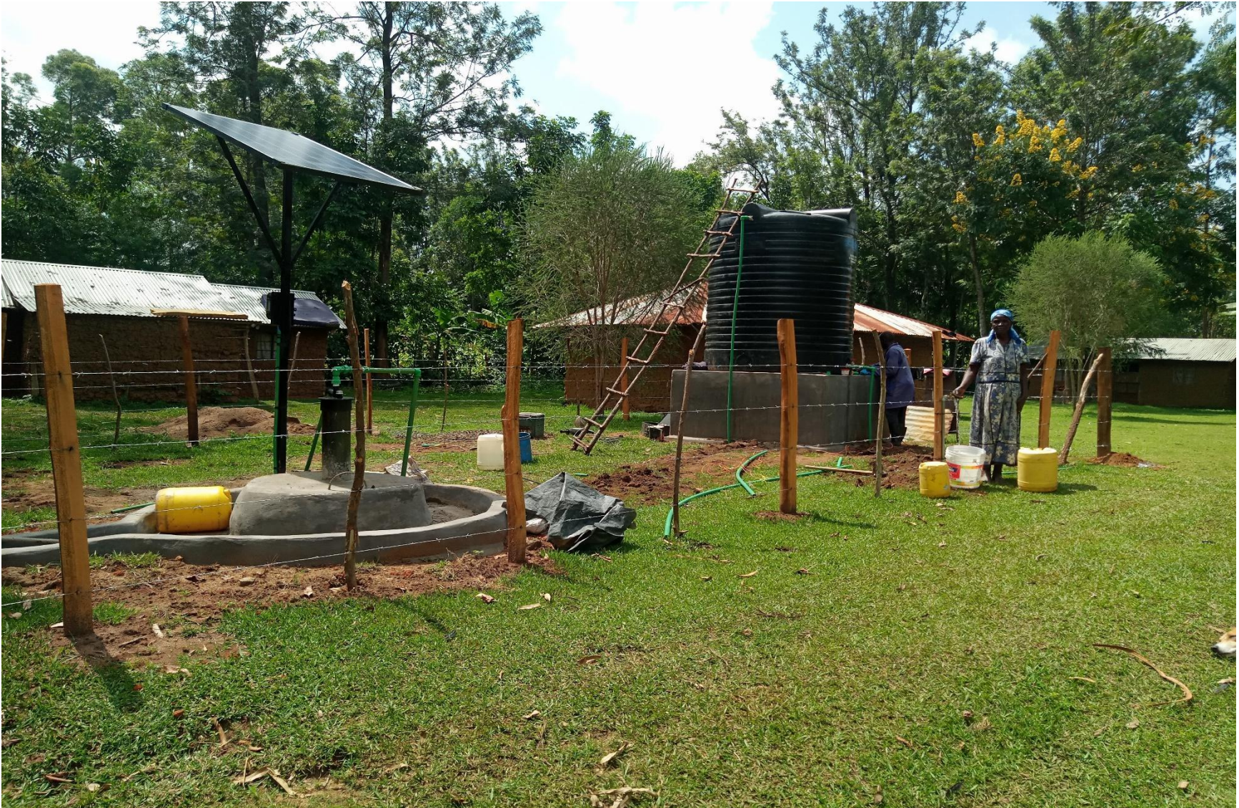
Lunao wajane women group shallow well installed with solar pumping system
