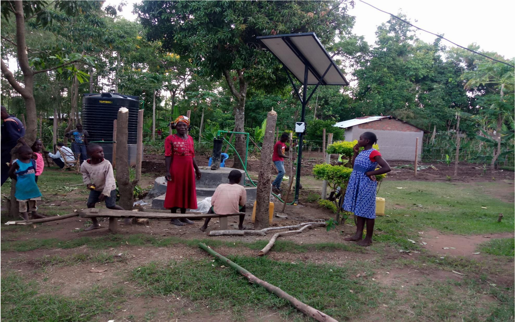
Siyengo Youth Group shallow well installed with solar pumping system.
