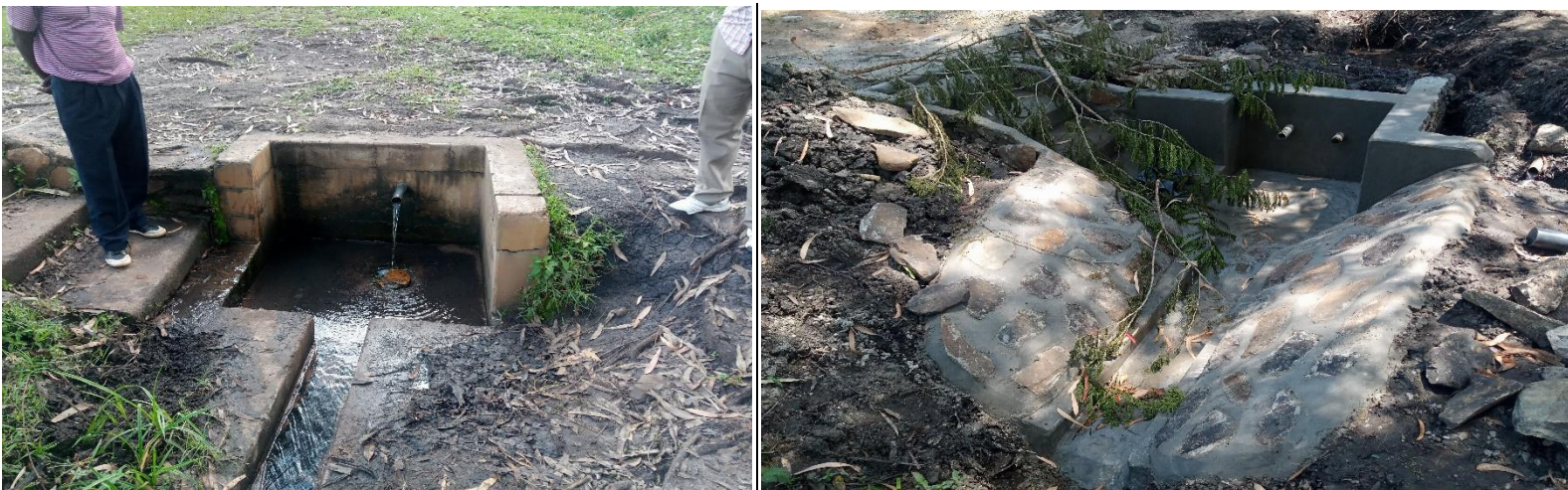
Namwetunde spring protection complete( Sio Sango Village)
