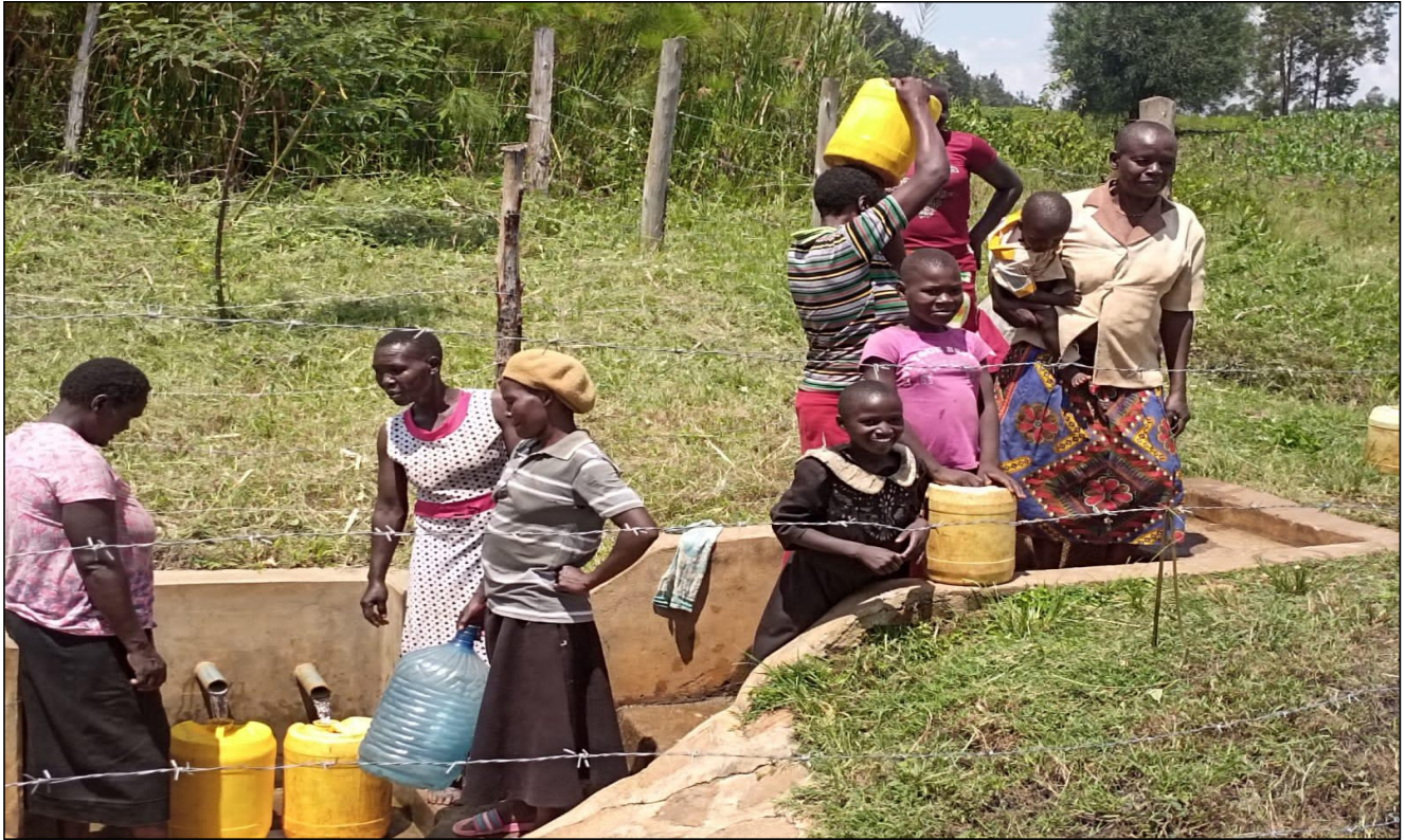
9.0 Completed Kibachenje Protected Water Spring in use by Community members
