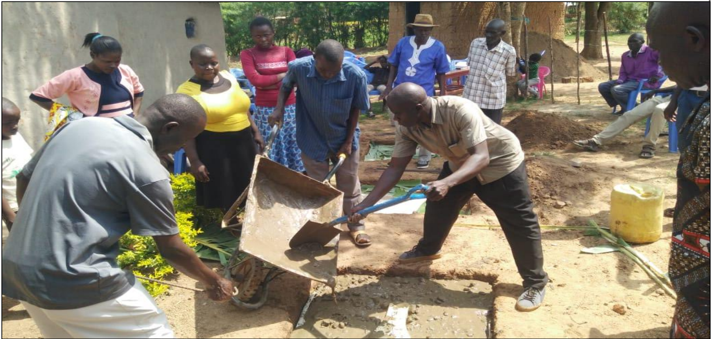
31.0 Community members participating in slab manufacture for Ecological sanitation/SANPLAT Households latrines development
