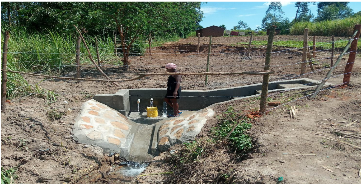
8.0 Completed Namusasi Protected Water Spring being used by Community members
