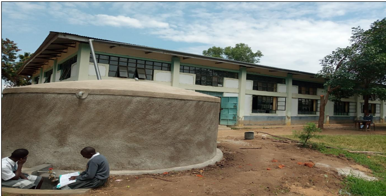
6.0 Completed 30,000litres Ferro-cement Water tank at St. Kizito Mayanja Secondary School
