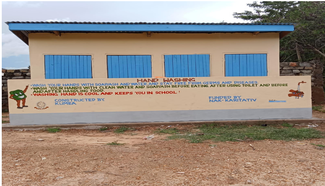
27. Completed 1no. 4door Ventilated Improved Pitl latrines at St.Joseph Bukurimo Secondary School
