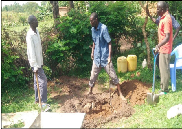
33.0 Preparing latrine pit & site for SANPLAT slab latrine construction
