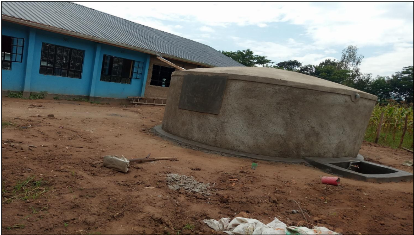
7.0 Completed 30,000litres Ferro-cement water tank for St. Peters Siboti Secondary School
