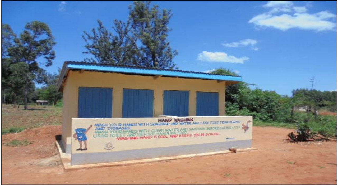
13.0 Completed 1no. 4door Ventilated Improved Pit latrines at Kimaeti Primary School
