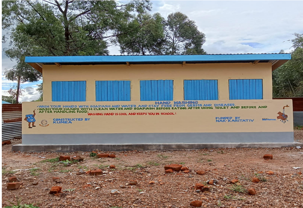
27.0 Completed 1no. 4door Ventilated Improved Pitl latrines at St.Kizito Mayanja Secondary School
