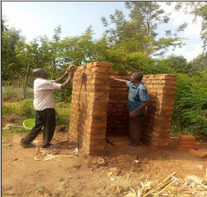
35.0 Superstructure latrine construction with bricks and mud mortar
