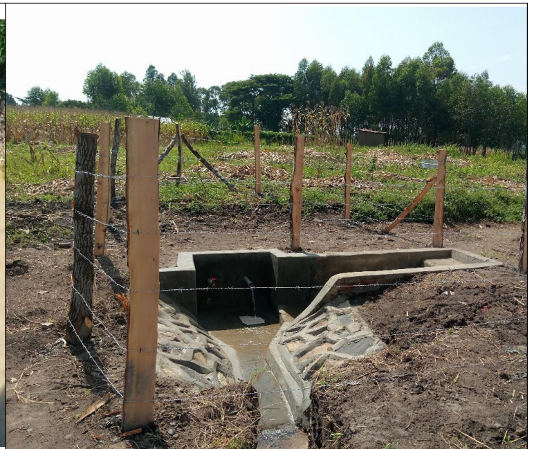
18B Munyolo Spring after construction & protection
