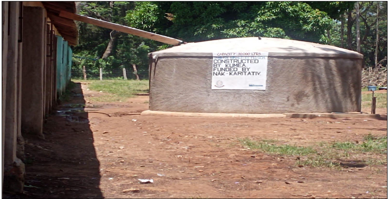
11.0 Completed Ferro-cement Water Tank at Kimaeti Primary School
