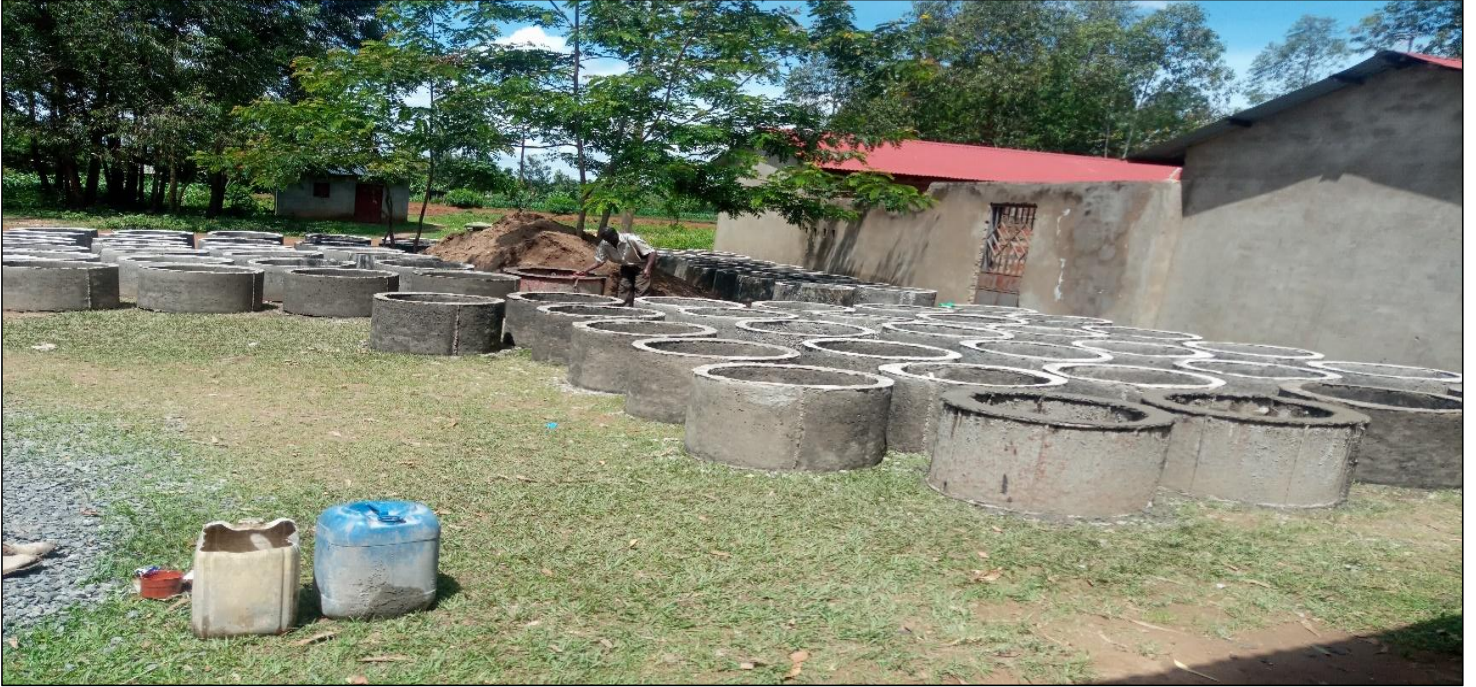
3.0 Manufacture & production of culverts for hand dug well construction and development
