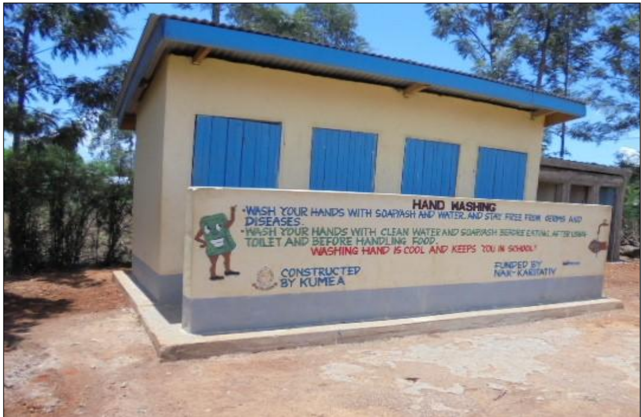
12.0 Completed 1no. 4door Ventilated Improved Pit latrines at Nakalila Primary School, Bumula Sub county
