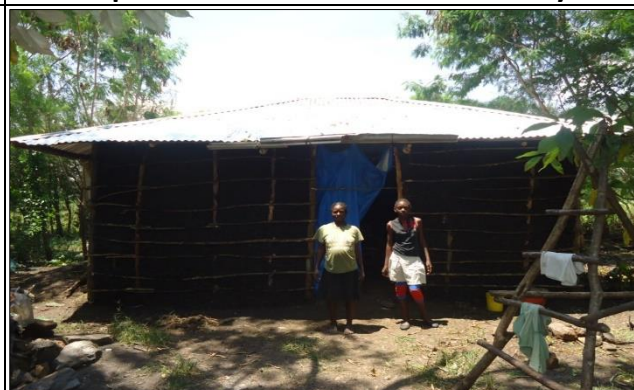
6. Completed house for vulnerable family –used mud &wattle for the walling
