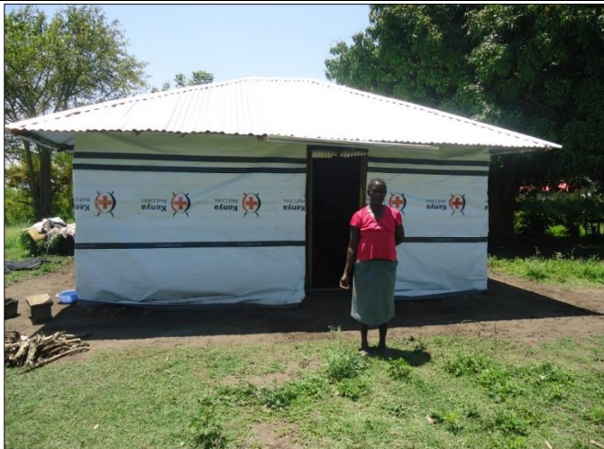
15. Completed house for vulnerable family
