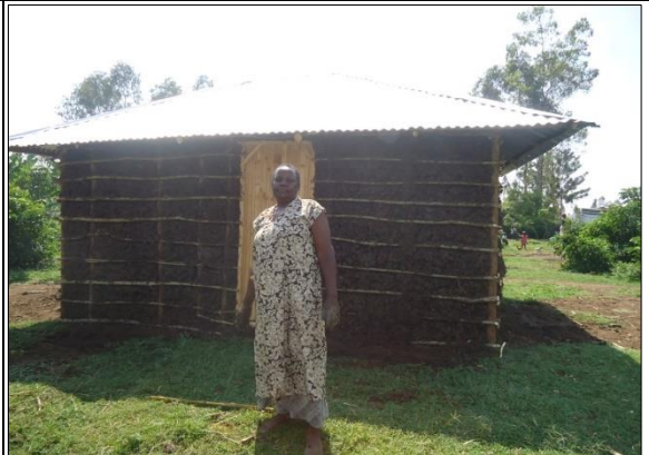
6. Construction of house completed with mud and wattle walls for vulnerable family
