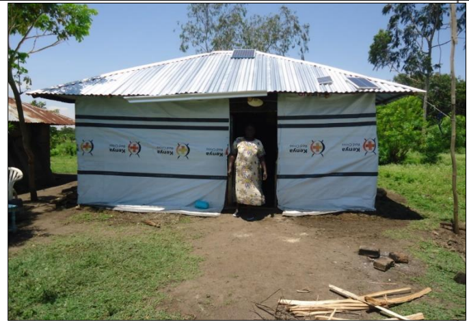
14. Completed house with canvas walling for vulnerable family
