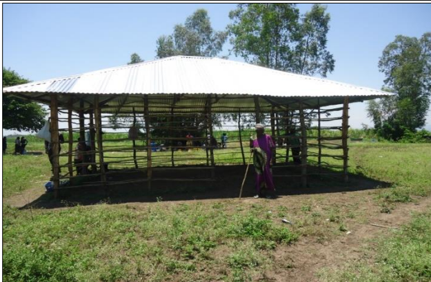
5. Partially completed house with roofing done
