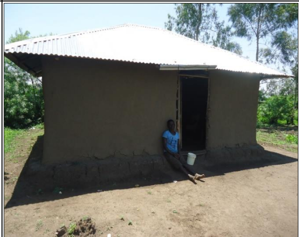
10. Completed house for single parent
