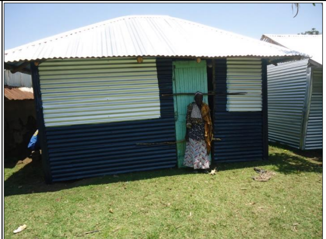
8. Completed house for elderly lady with iron sheets roofing & walling
