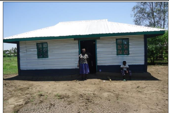
12. Completed house for single parent
