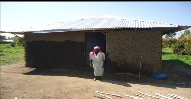
17. Completed house for the elderly & vulnerable family
