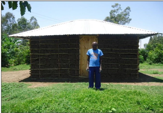
13. Completed house for vulnerable family
