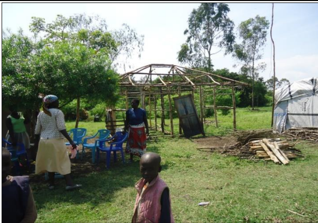
3. Construction of houses and shelters on-going
