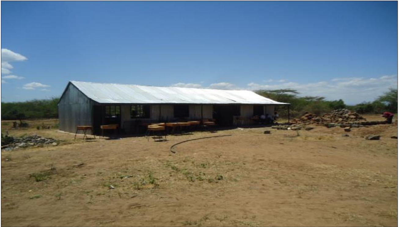
1. Completed classrooms at Salabani mixed Secondary school with support of the project
