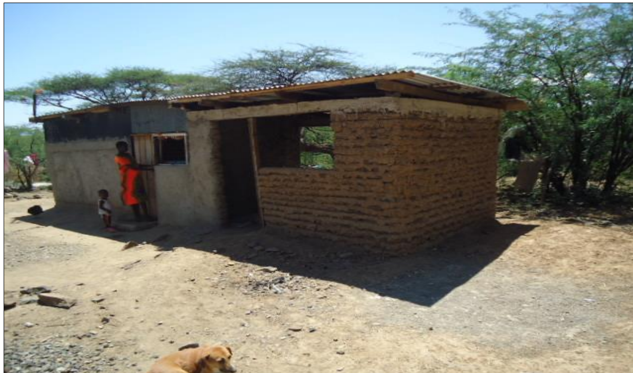
11. House under construction in Kipkimbirwo village
