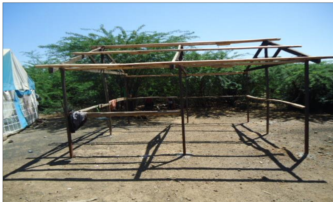
12. House under construction in Kipkimbirwo village
