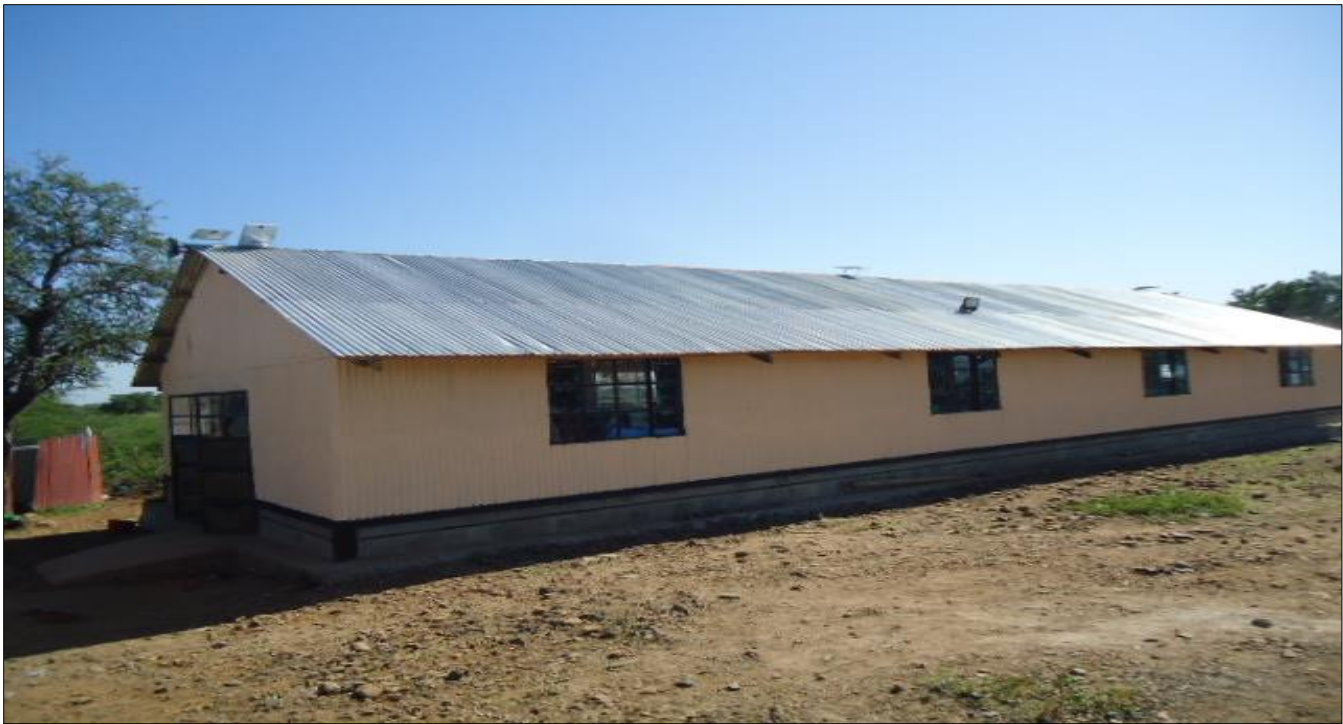
4. Completed boys' dormitory for Lake Baringo Mixed Secondary school with support of the project
